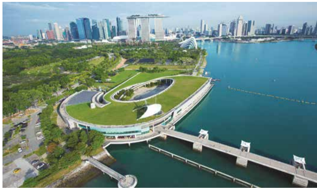
The Marina Barrage creates a freshwater reservoir in the heart of the city
