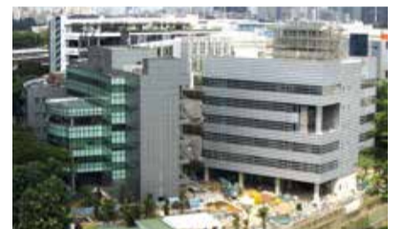
Singapore Water Exchange
